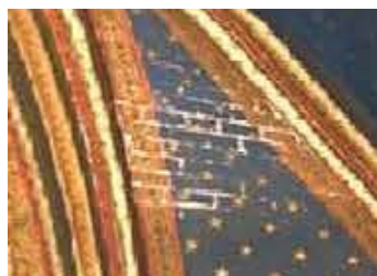
Close-up view of damage caused by past leaks, and a medallion
